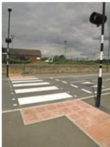
Pedestrian crossing improvement at Belper.
